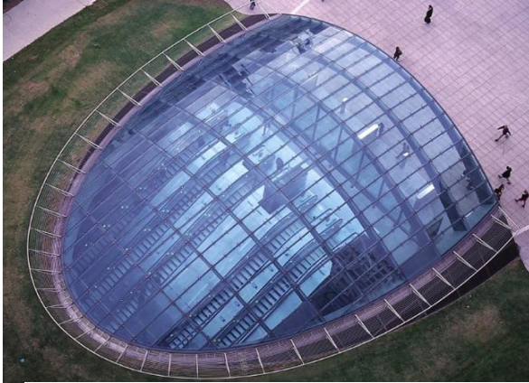
Figure 1: canopy of subway entrance
