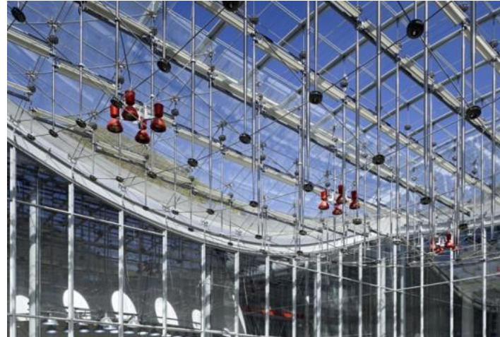
Figure 5: skylight embraced into the roof
